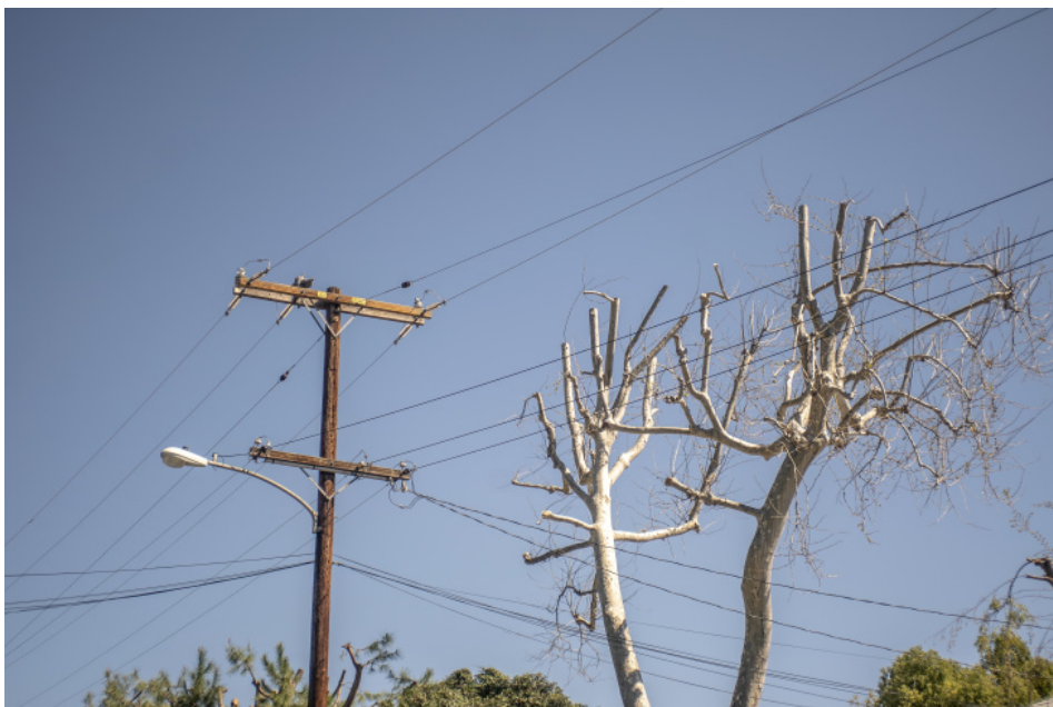
California Edison is trimming trees in Altadena angering residents who believe the power company is going too far. (Chava Sanchez/ LAist)
